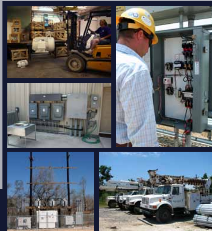
Pictured on center fold from top left: 1. REI's electrical motor stock, 2. Commercial building power distribution, 3. Troubleshooting & repairing electrical work, 4. Saltwater Disposal Power System, 5. Poleline construction equipment
